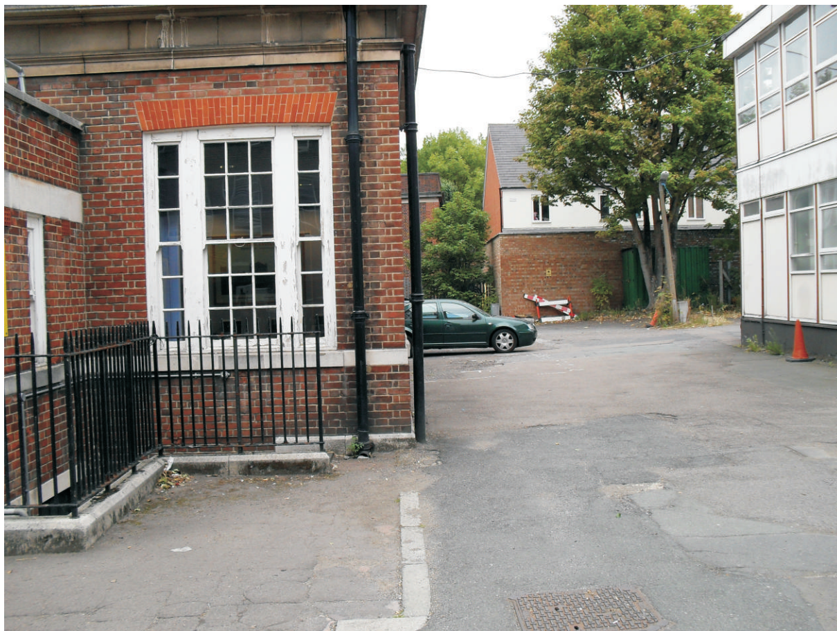
Plate 15: East facing photograph of 'The Clinic'
