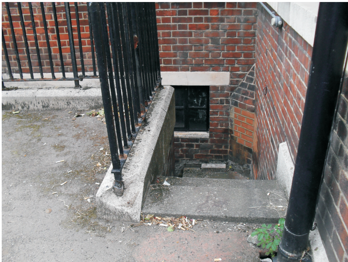
Plate 17: North facing photograph of access to 'The Clinic' basement
