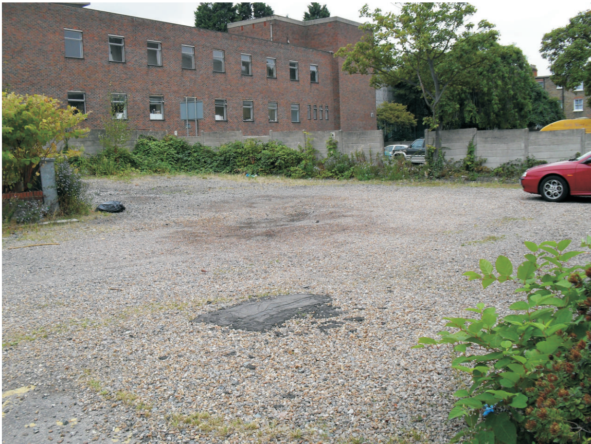
Plate 13: South west facing photograph of gravel car park with library car park in background
