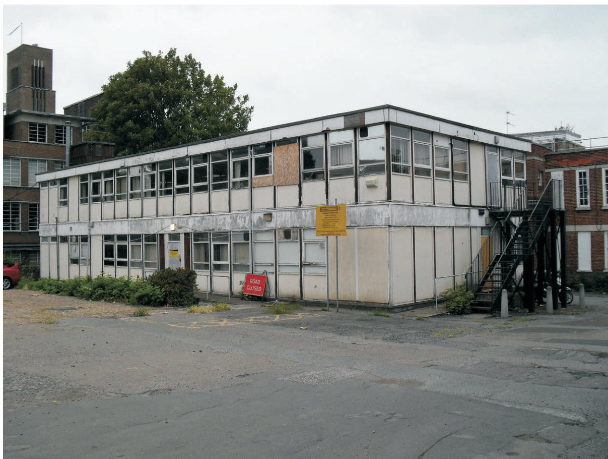
Plate 8: North West facing photograph of 2 storey 1970s 'pre-fab' building
