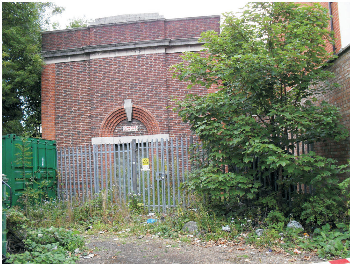
Plate 9: East facing photograph of electricity sub-station
