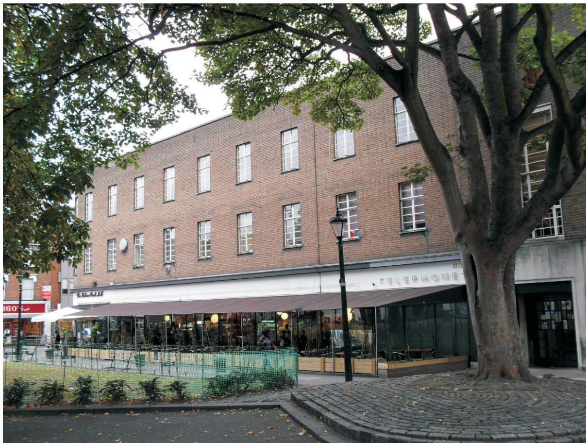
Plate 11: North west facing photograph of former Electricity Showroom (now Broadway Annexe)
