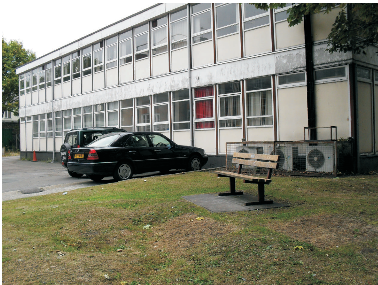
Plate 16: South east facing photograph of 'pre-fab'
